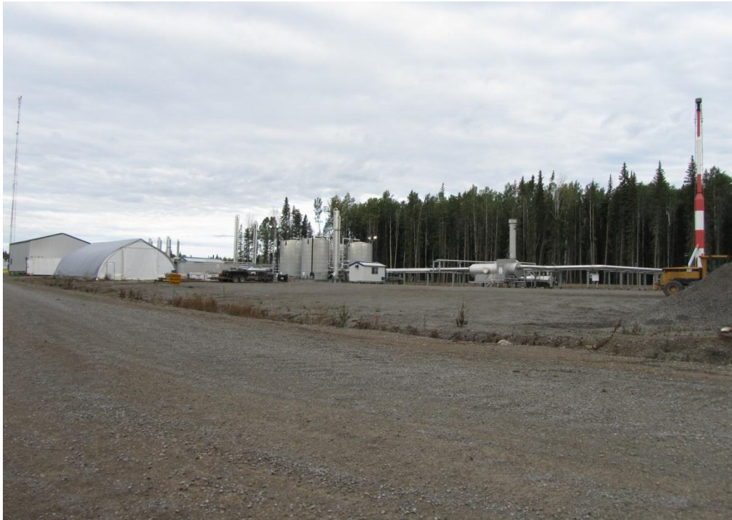
Fig 1b. Oil and Gas Facilities at Quick Silver
